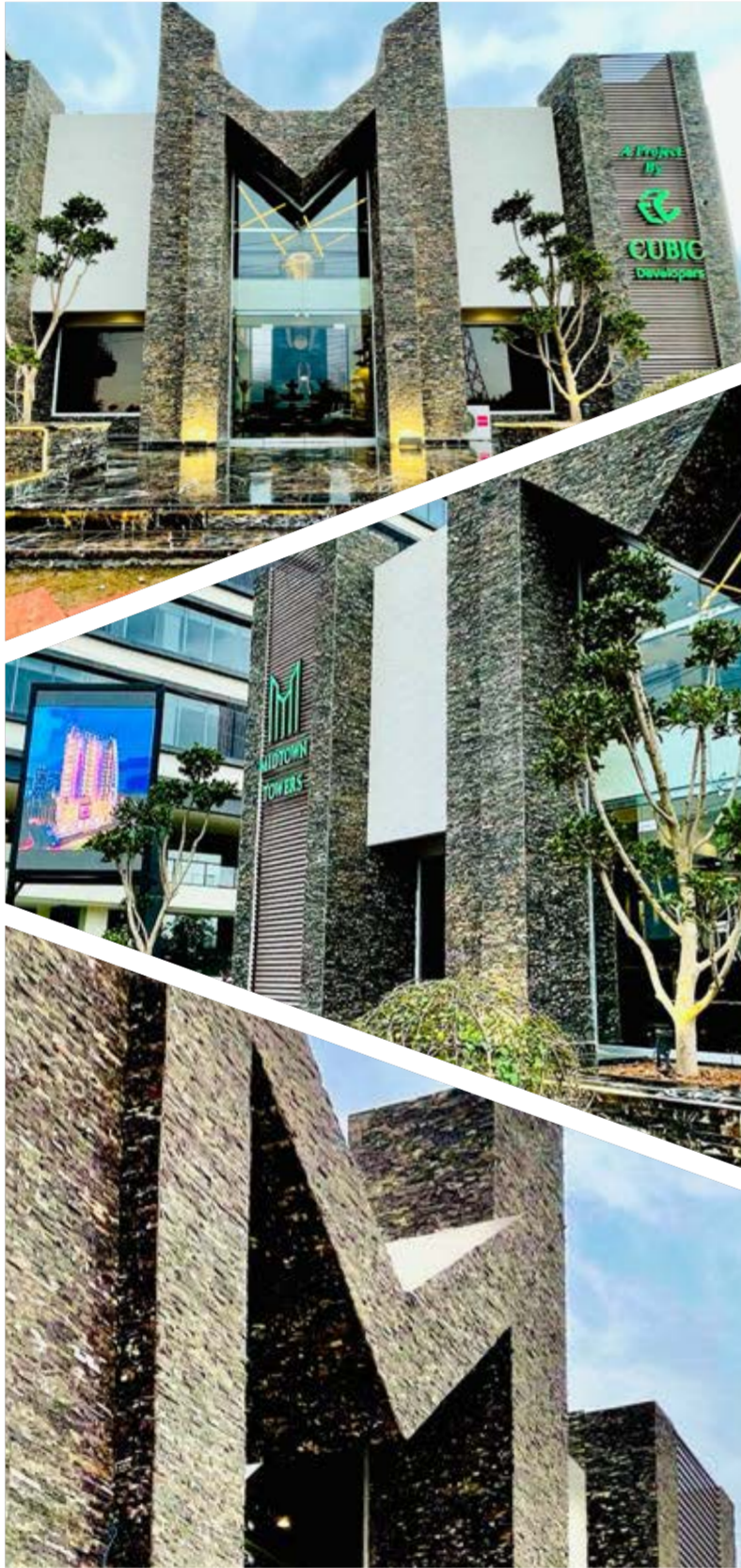
MIDTOWN TOWERS SITE OFFICE H-13
